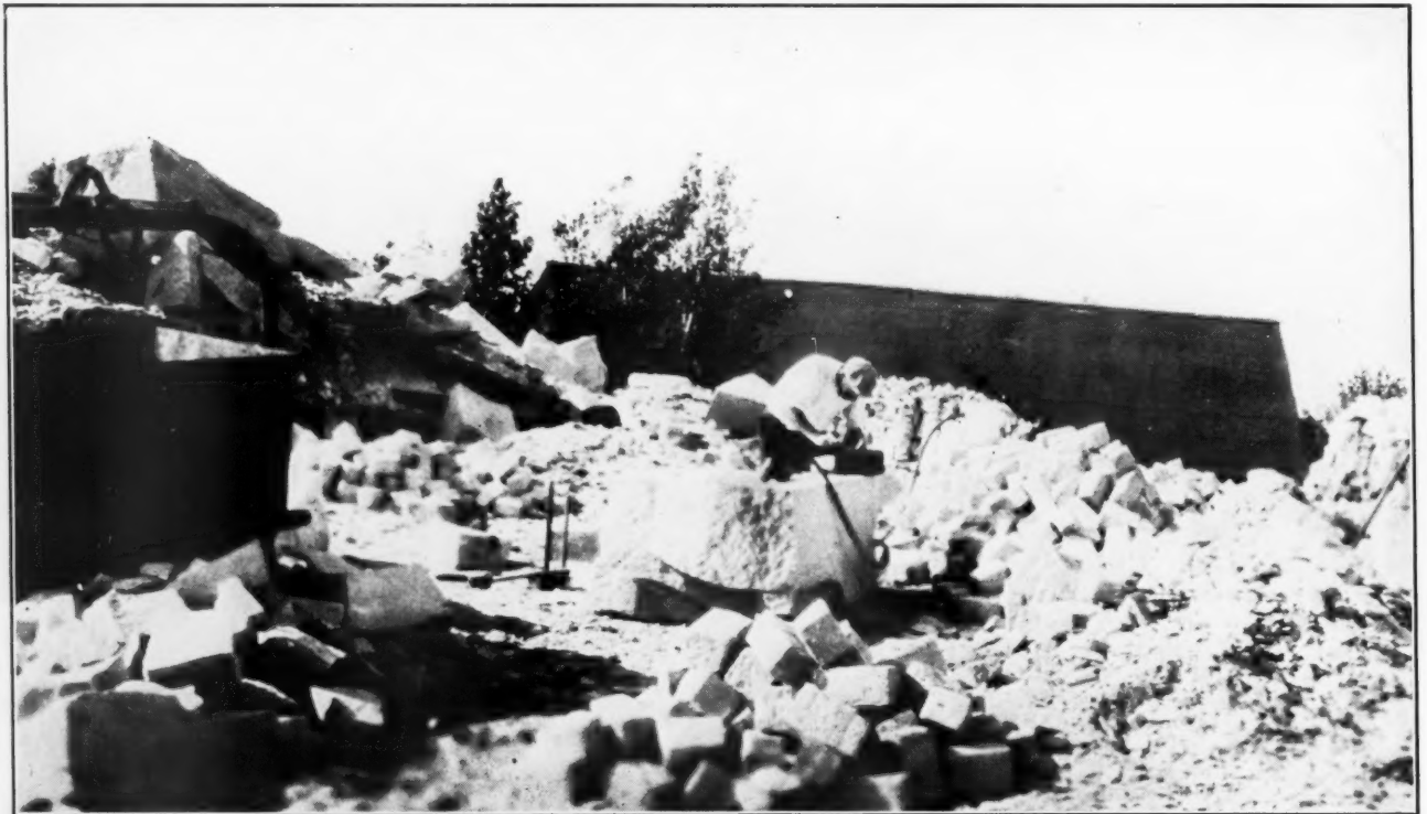
Upper Left—Part of the Quarry and Derricks. Upper Right—Elevator from Crusher to Cylindrical Screen. Note box made of old boiler section filled with stone ready to dump into crusher. Lower—Making paving blocks with the help of small drills
